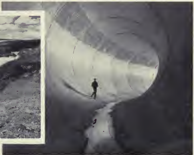
SOOP LAKE SIPHON (below) outside view. At lower right, inside the Soop Lake siphon, a 25-foot-diameter tube, 2½ miles long. Both photos by H. E. Foss, Region 1.
